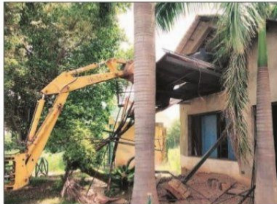
GMADA removes illegal constructions in Mohali. Express
